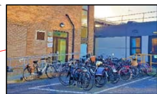
CUTRTO - Norman Bleehan Offices
